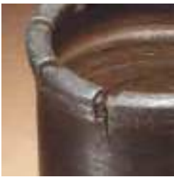
CRACKS IN THE WATER WAYS
